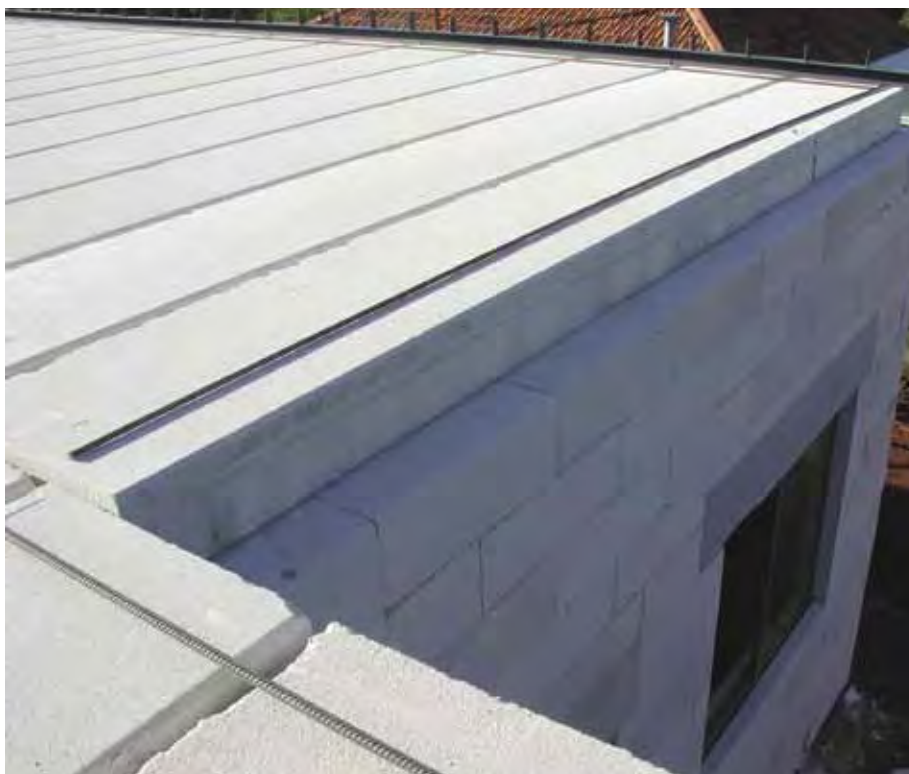
Image 7.3.2: Installed Floor Panels
